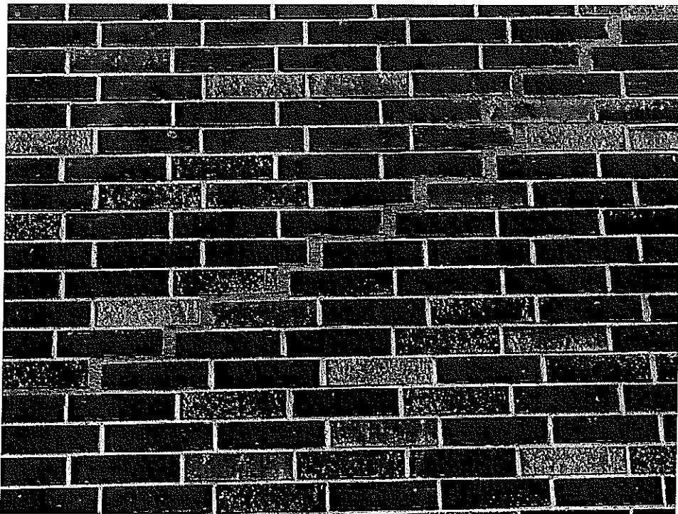
Figure 9 – Typical brick repairs (bldg 15).
